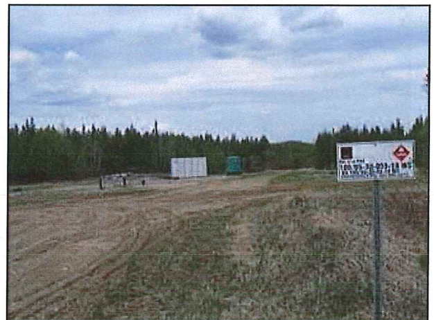
(Right) Wellsite near SE Corner of Block 2 Parts of Blocks 2 and Block 3 to the East were taken out by the construction of this wellsite and pumping station. The road forms the boundary between the blocks. Photopoint 1 is in the SW corner of the wellsite, Photopoint 2 just off the NW corner.
