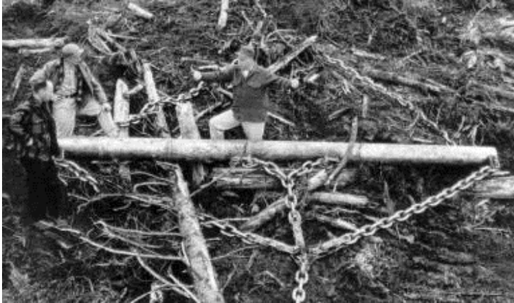
CHARLEY JACKSON (AFS), REG LOOMIS (AFS) AND DES CROSSLEY EXAMINE EARLY SCARIFICATION DRAG AND SPREADER BAR, LATE 1950S WELWOOD PHOTO COLLECTION
