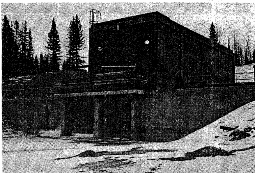
Pump house intake.
