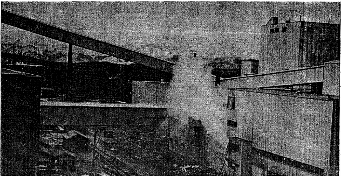
Steam and power plant with recovery group on the right.
