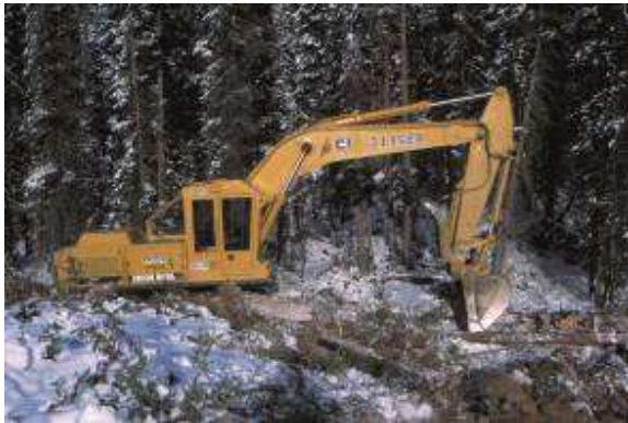
Excavator Mounding on Wet Sites
