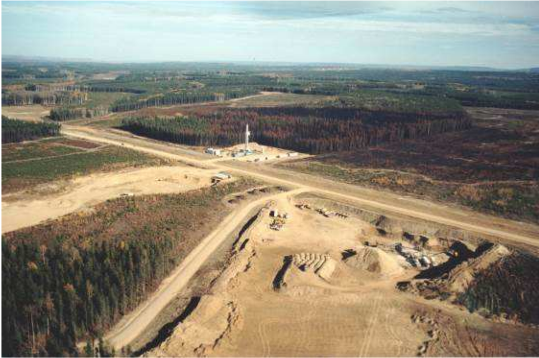
GAS FIELD DEVELOPMENT NORTH OF HINTON, 2004.
