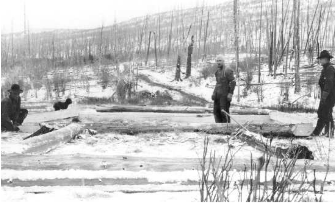
FIRE WAS NO STRANGER TO THE EASTERN SLOPES, AS CAN BE SEEN IN THIS PICTURE OF THE MOBERLY CABIN CONSTRUCTION, 1939. IN THE BACKGROUND ARE FIRE KILLED SNAGS FROM THE FIRES OF THE 1880S
