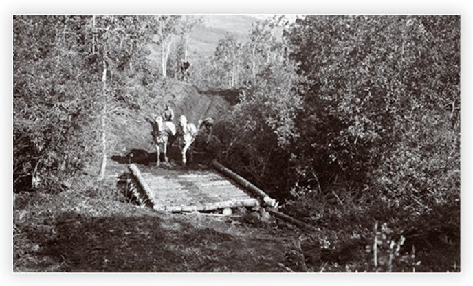
The early Forestry bridges, such as the ones across the Wildhay and Berland Rivers, were typically built of local timber with log abutments and rock-filled cribs to support longer spans. The bridge in this photo is on the Highwood-Pekisko Creek road in the Bow River Forest, 1923.
