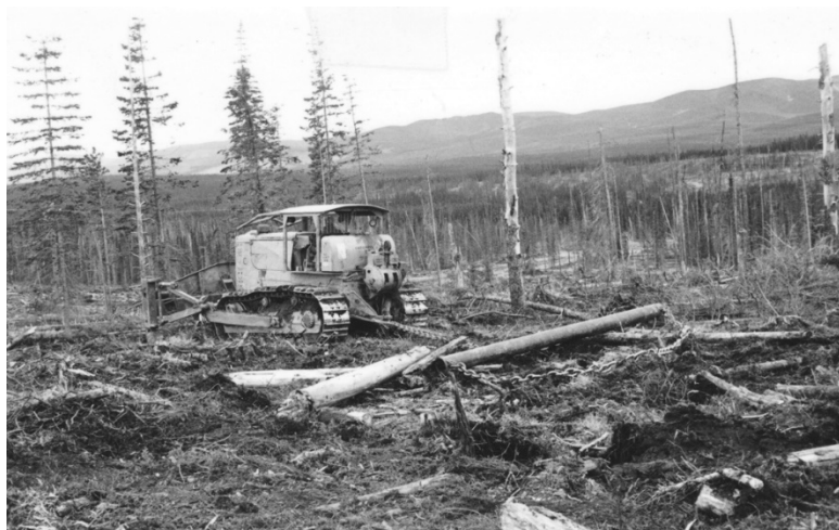
First anchor chain drag, a loop of chain behind the spreader bar.
