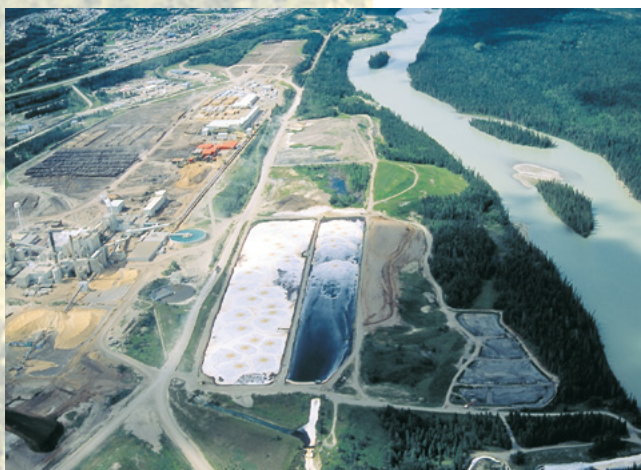
Treatment ponds aerate effluent from the pulp mill and sewage from the Town of Hinton to reduce biochemical oxygen demand in the discharge.
