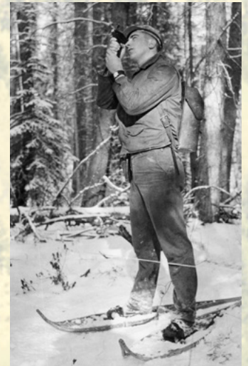
Timber cruiser Pete Dzwenko uses a Haga altimeter to measure tree heights on a CFI plot in 1963. Note the use of a tape recorder to record tree information, an innovation pioneered by NWPP.
