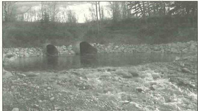
Restoration of fish passage through Hardisty Creek culverts
