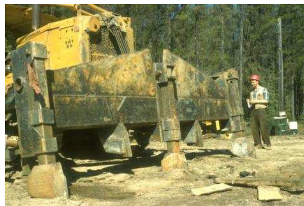
Early scarification equipment: Flecco Rake (l), 1956 and scarification plough on D9 tractor (r) 1959 with Forester Owen Bradwell
