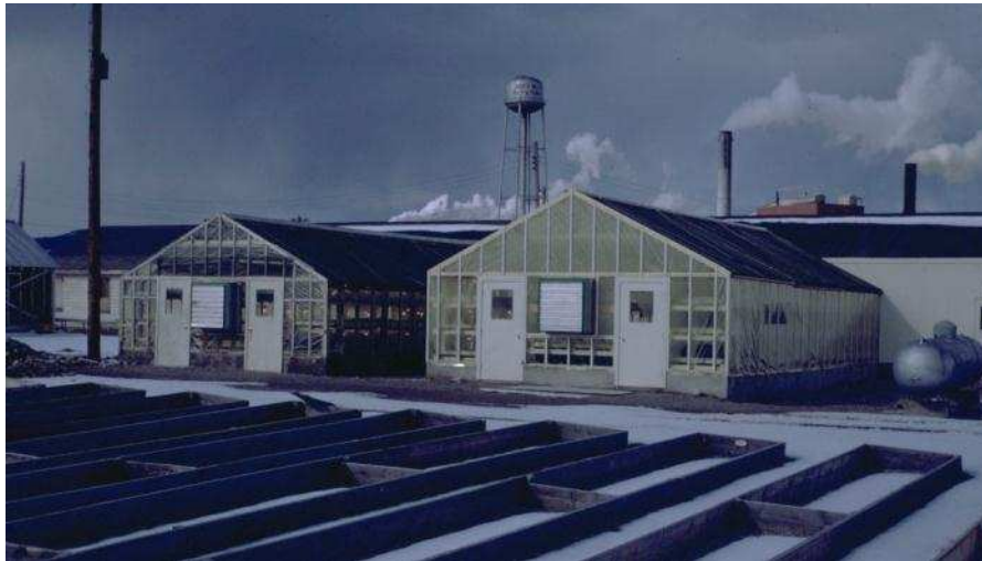
Greenhouses, 1968 HINTON WOOD PRODUCTS COLLECTION
