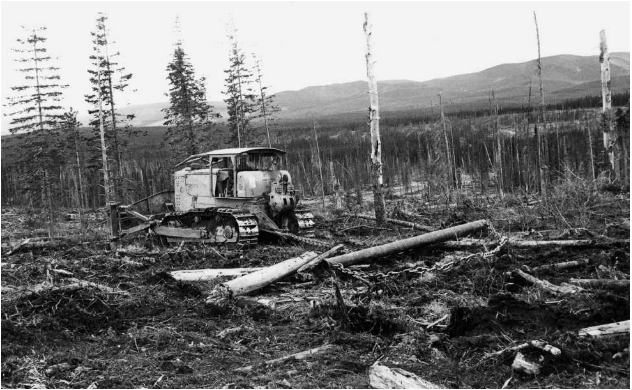
An early approach to scarification using a rudimentary chain drag
