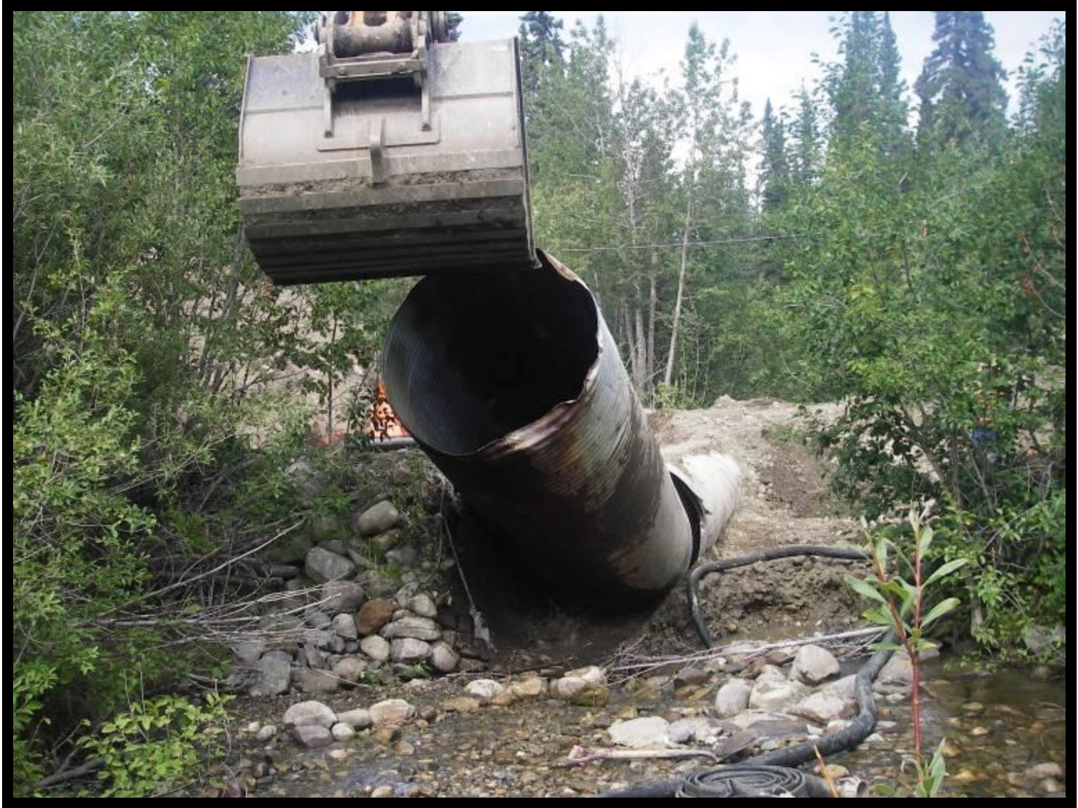
Removal of the culvert
