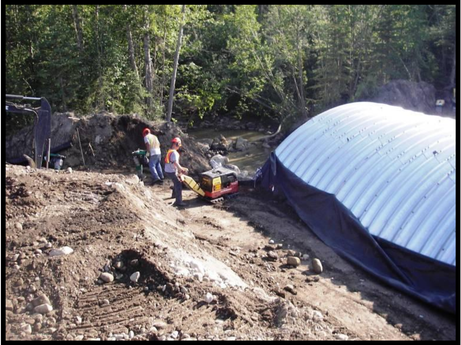
Compaction of soil around the arch
