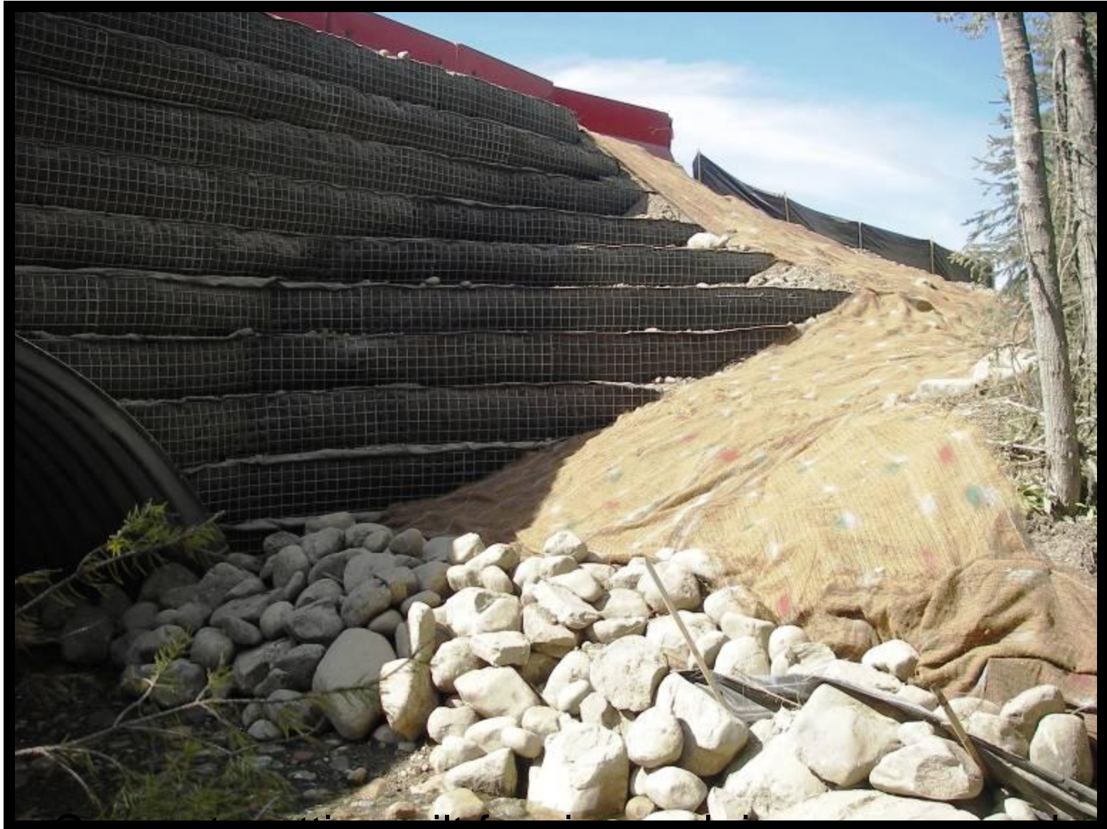
Coconut matting, silt fencing and rip rap was used as sediment control at the outlet
