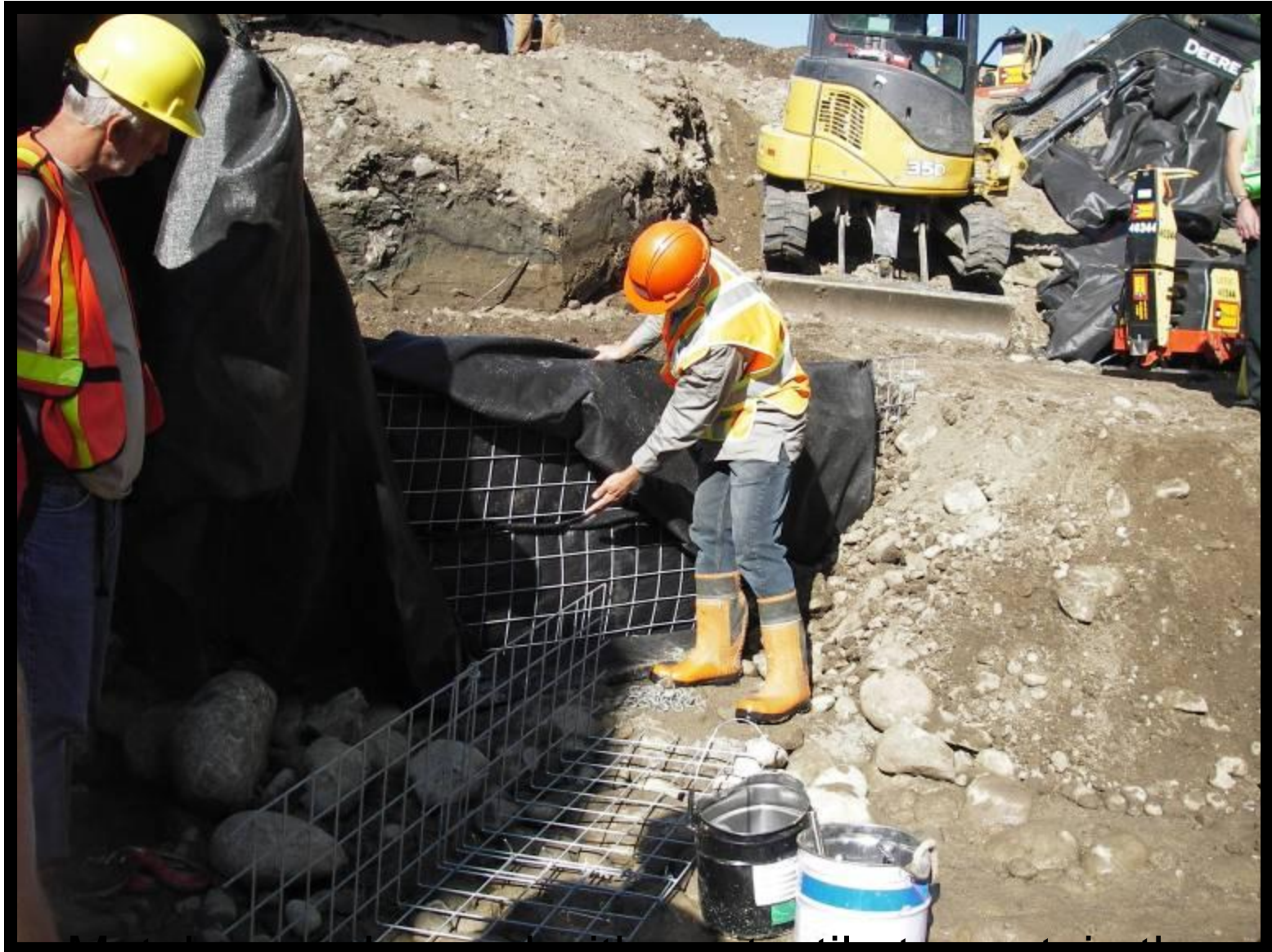
Metal cages layered with geotextile to contain the compacted soil
