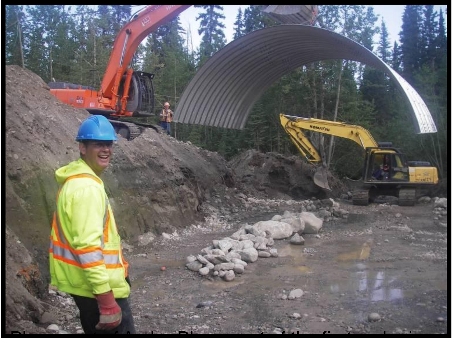
Placement of Arch - Placement of the first arch piece into the streambed
