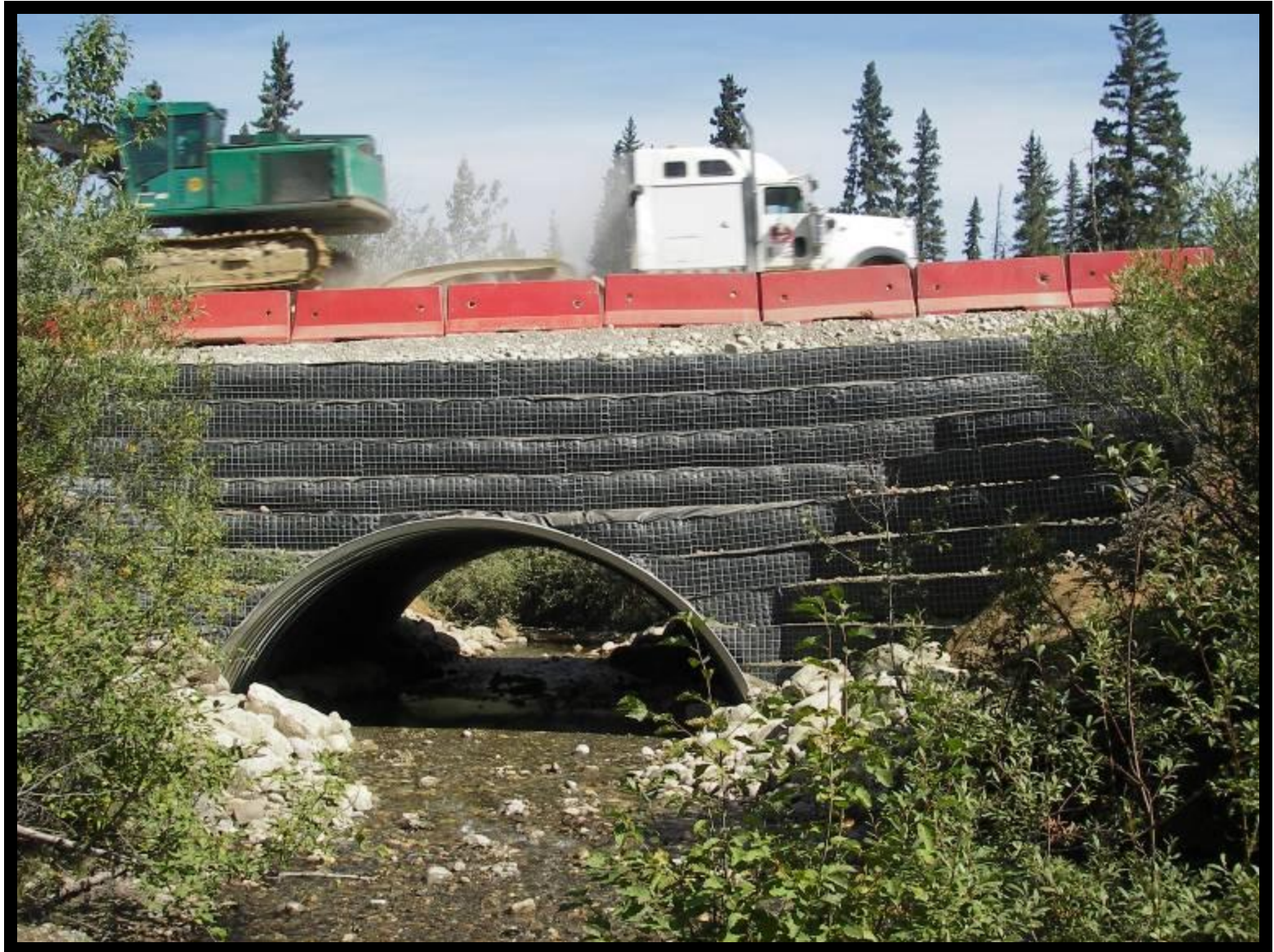
View of inlet as a semi-truck passes over
