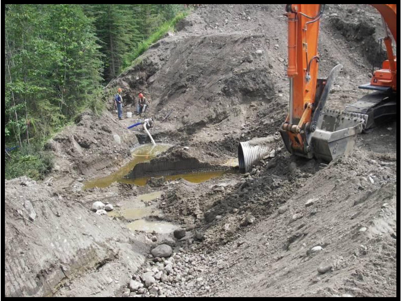
Removal of the culvert
