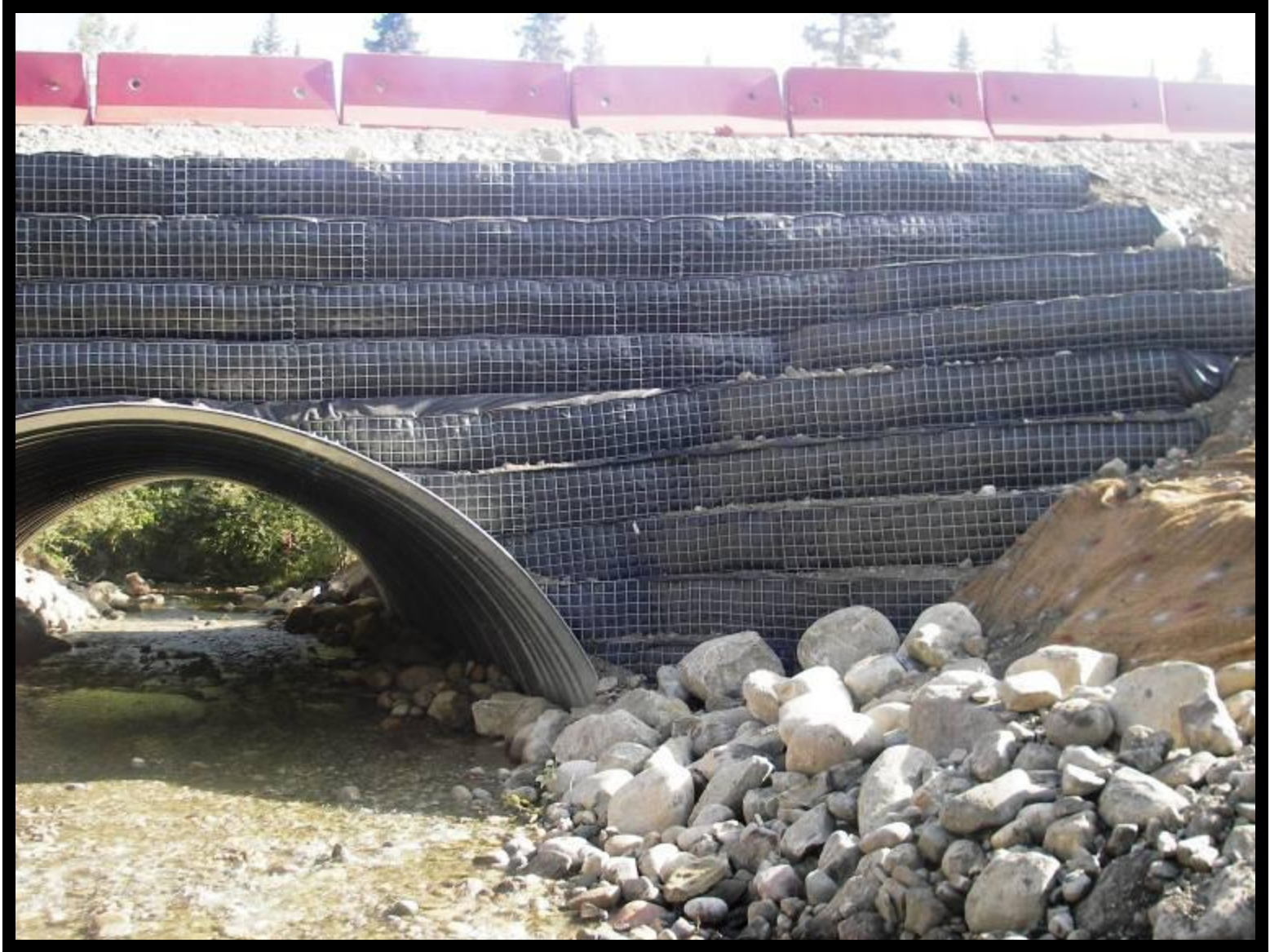
Inlet - View of inlet
