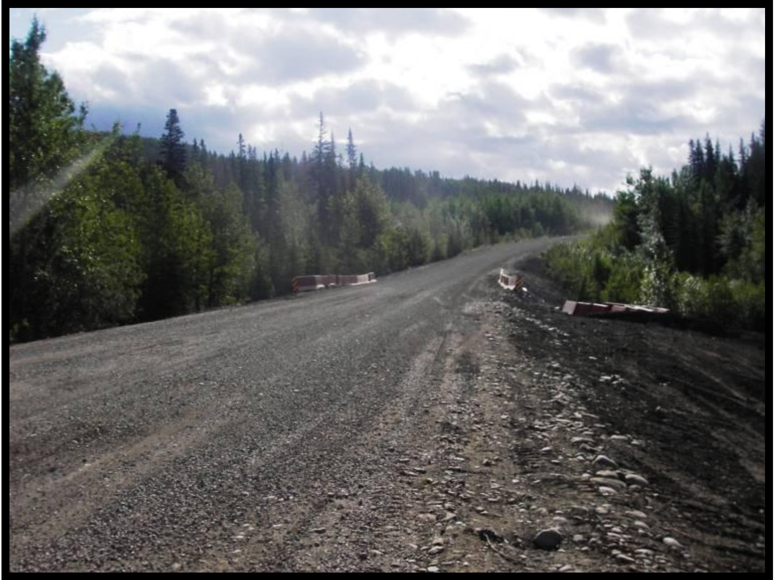
View of the road after construction
