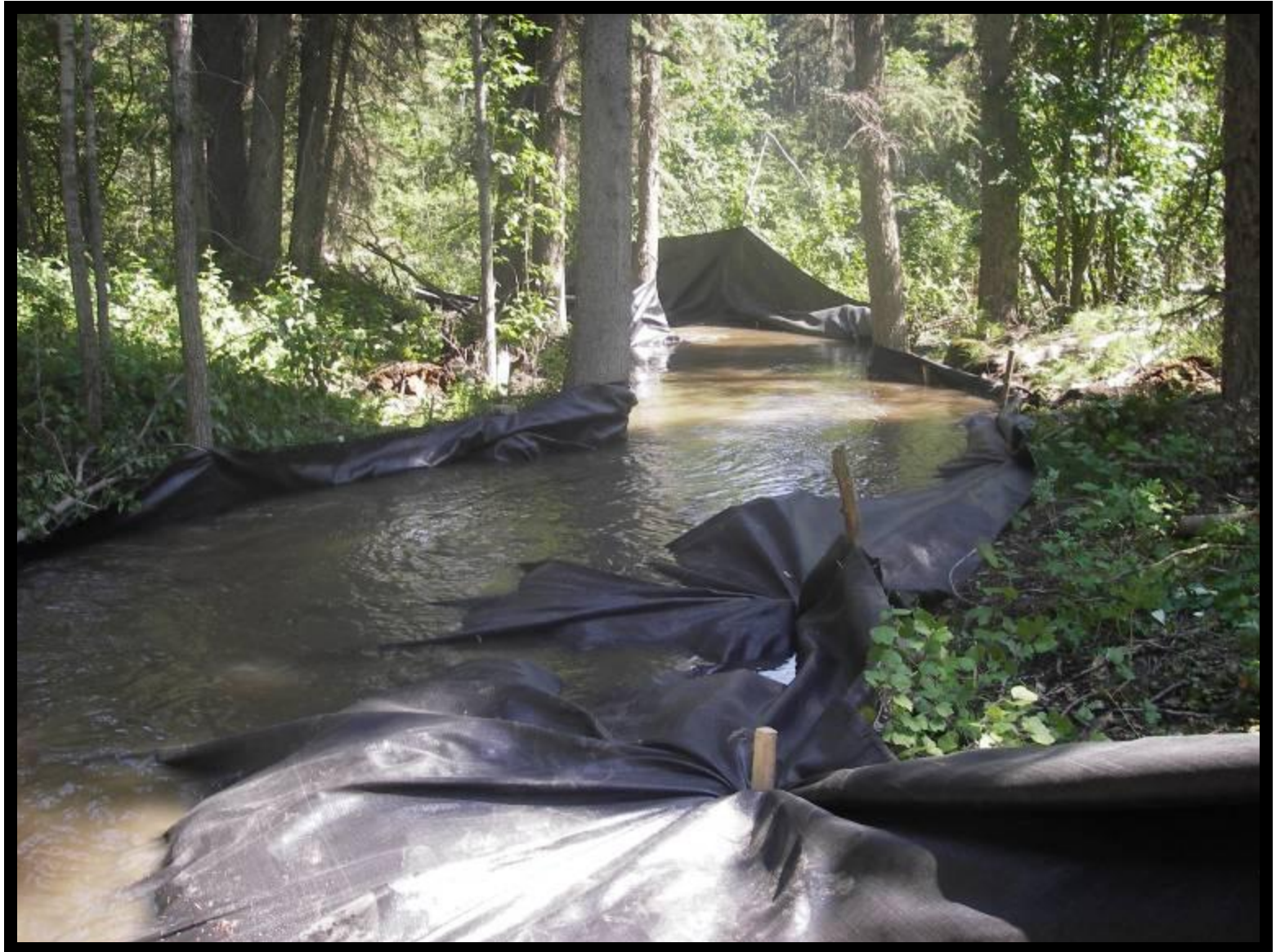
Downstream diversion ditch in action
