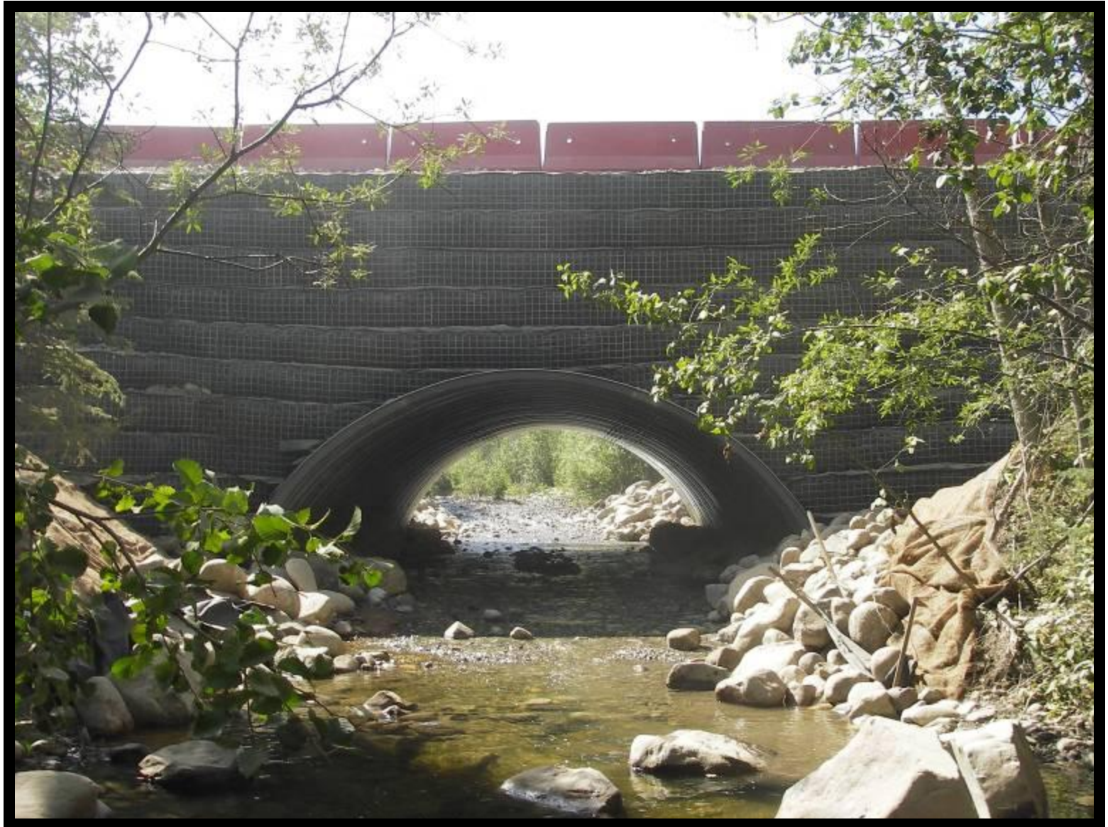
Outlet - View of outlet after construction
