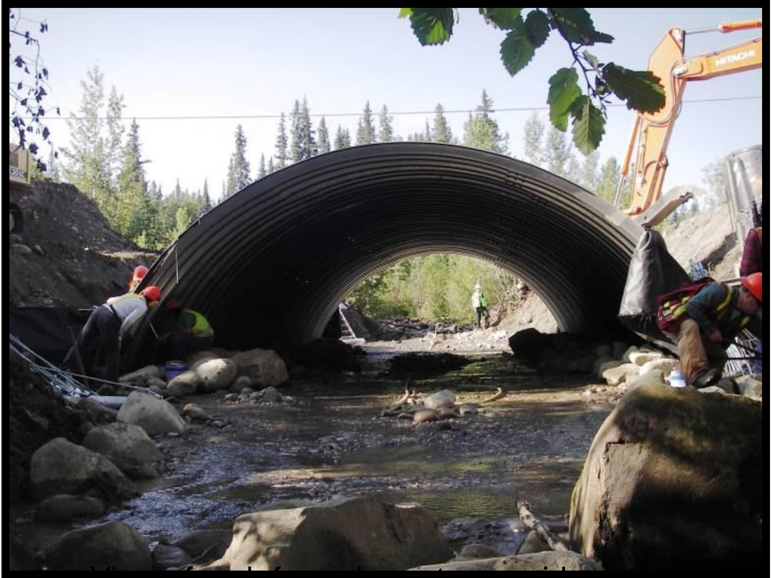
view of arch from downstream side during construction
