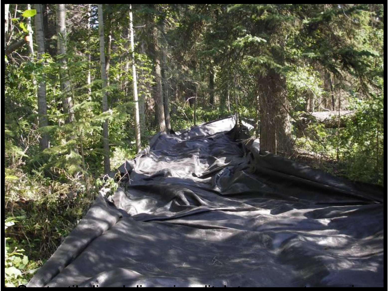
Geotextile lined diversion ditch to prevent scouring of forest floor
