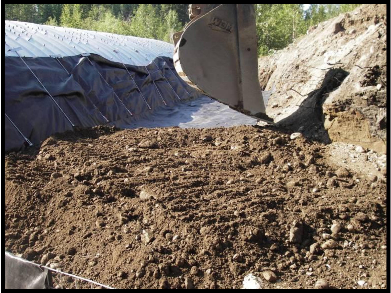
Compaction of soil around the arch
