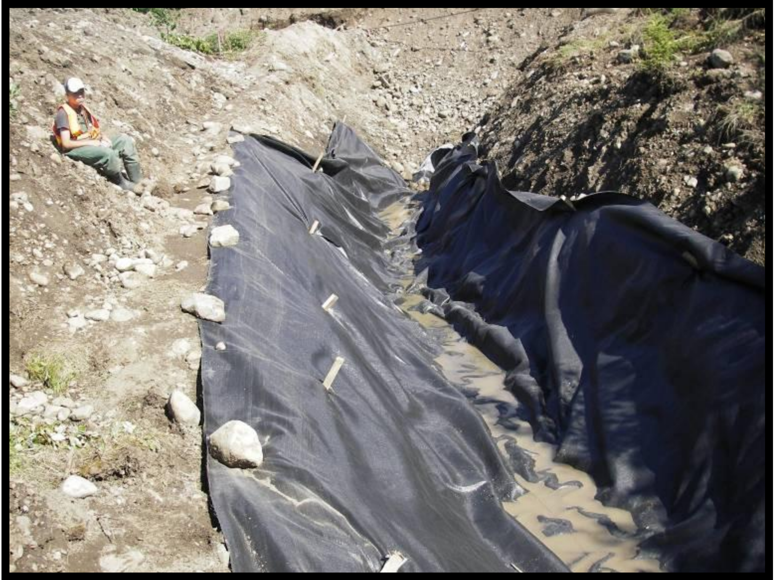
Stream diversion ditch upstream
