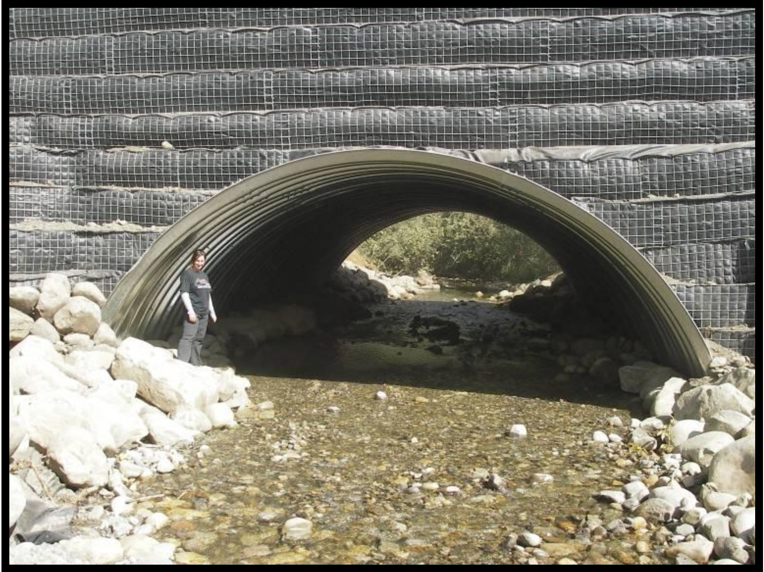
Inlet - Arch inlet after completion of construction
