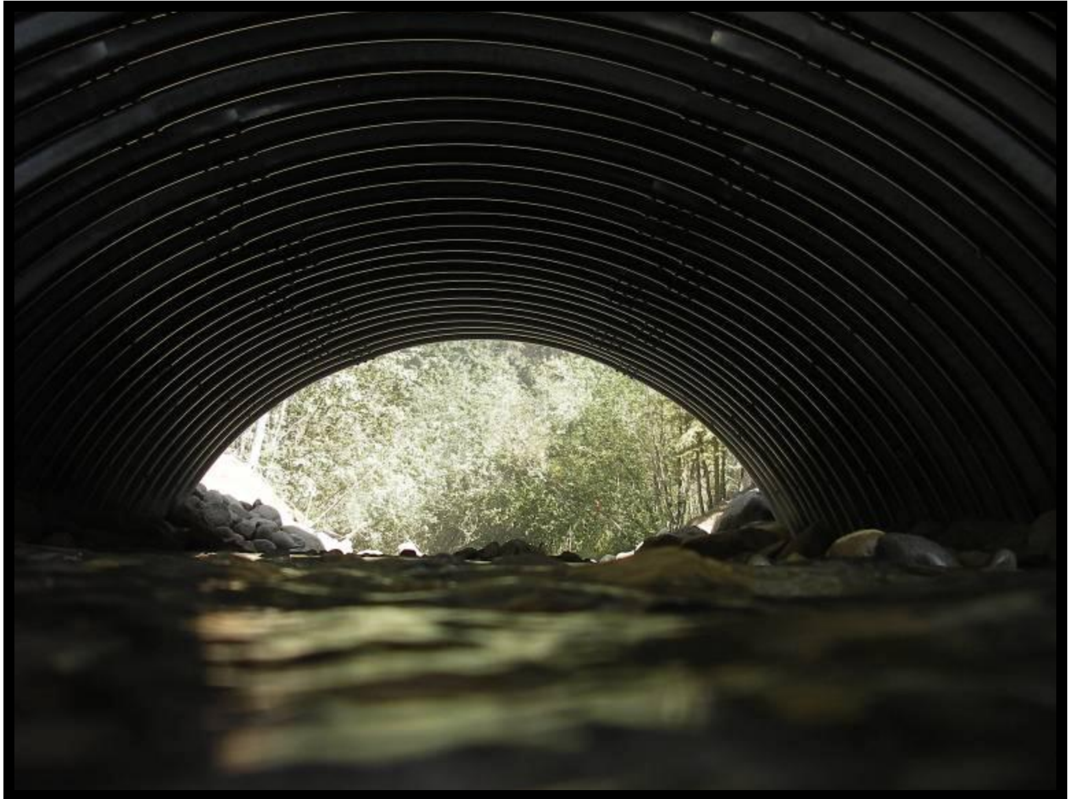
View of arch from water level facing downstream
