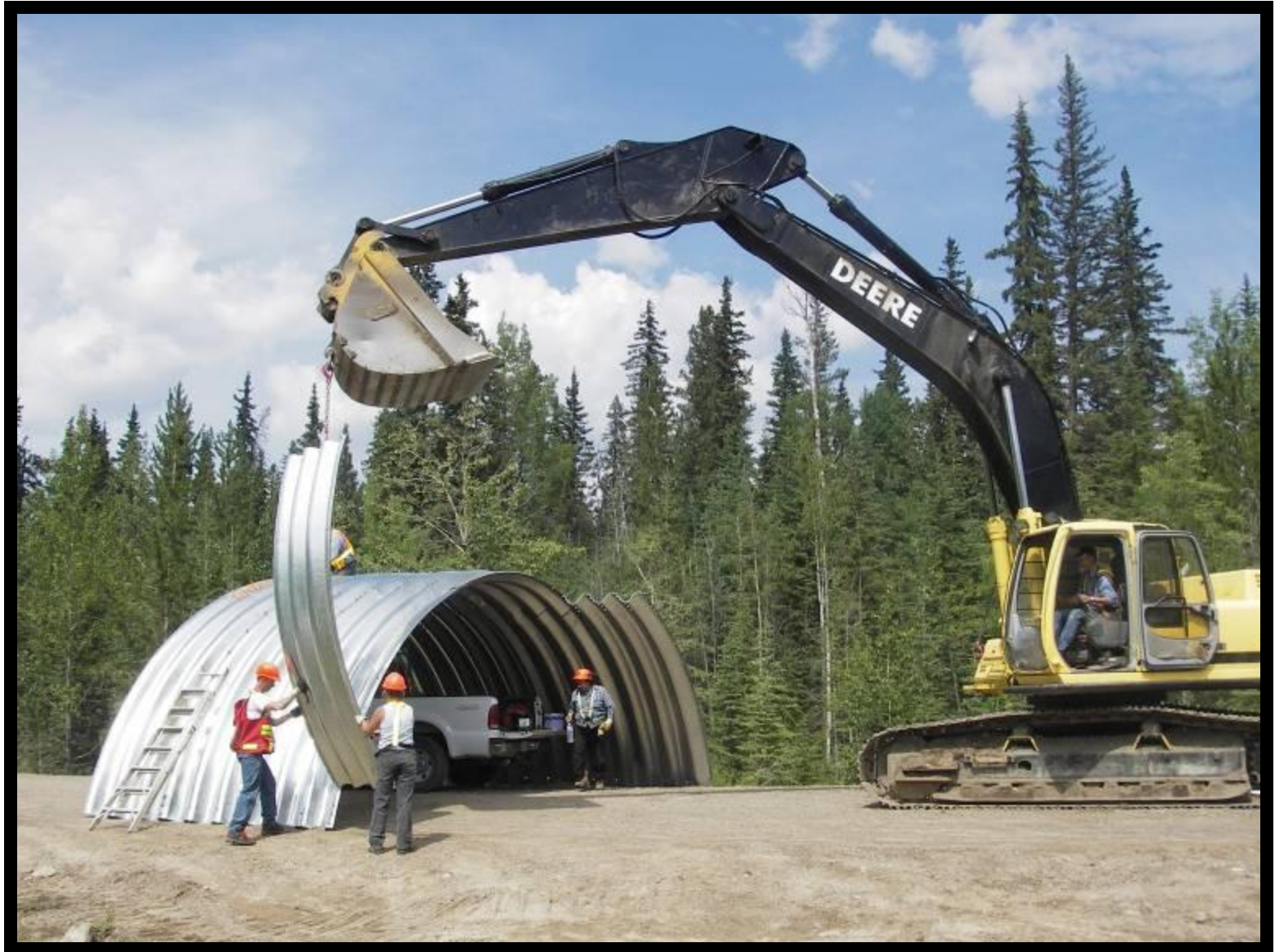
Construction of the metal arch
