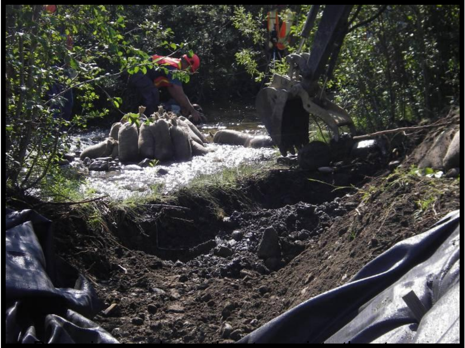
Preparing to release the stream into the stream diversion ditch
