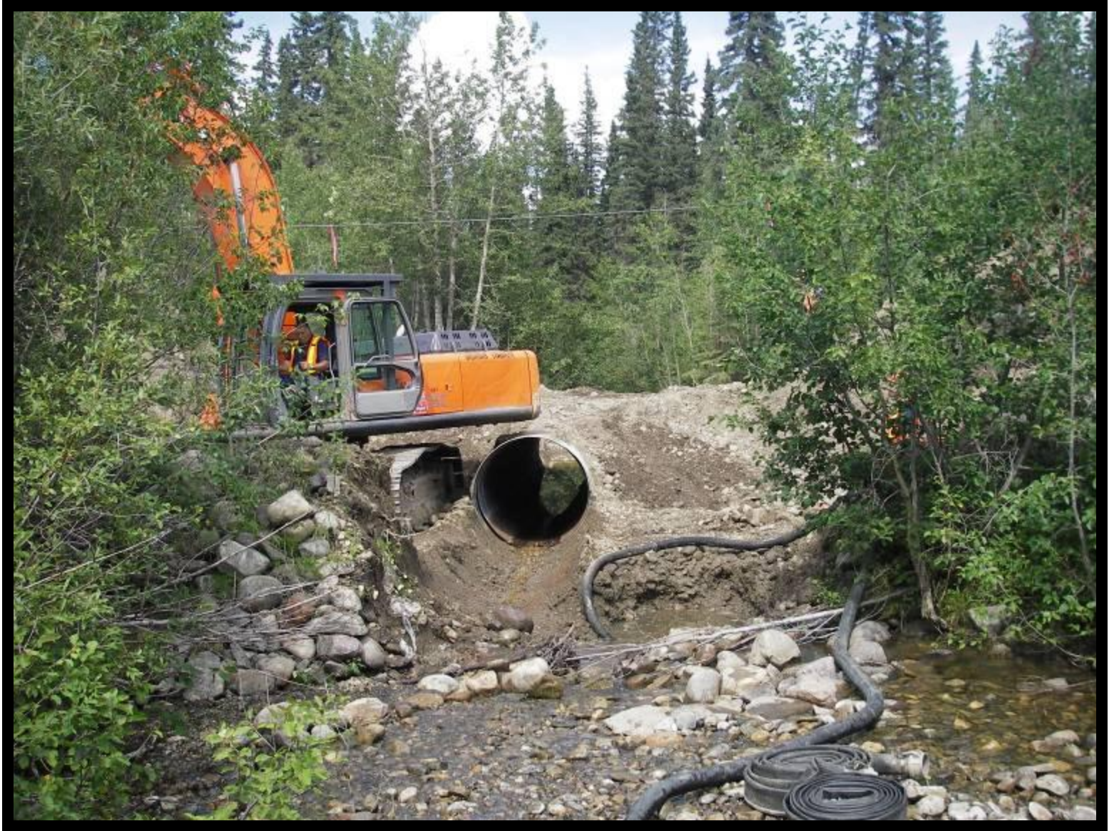
Removal of the culvert
