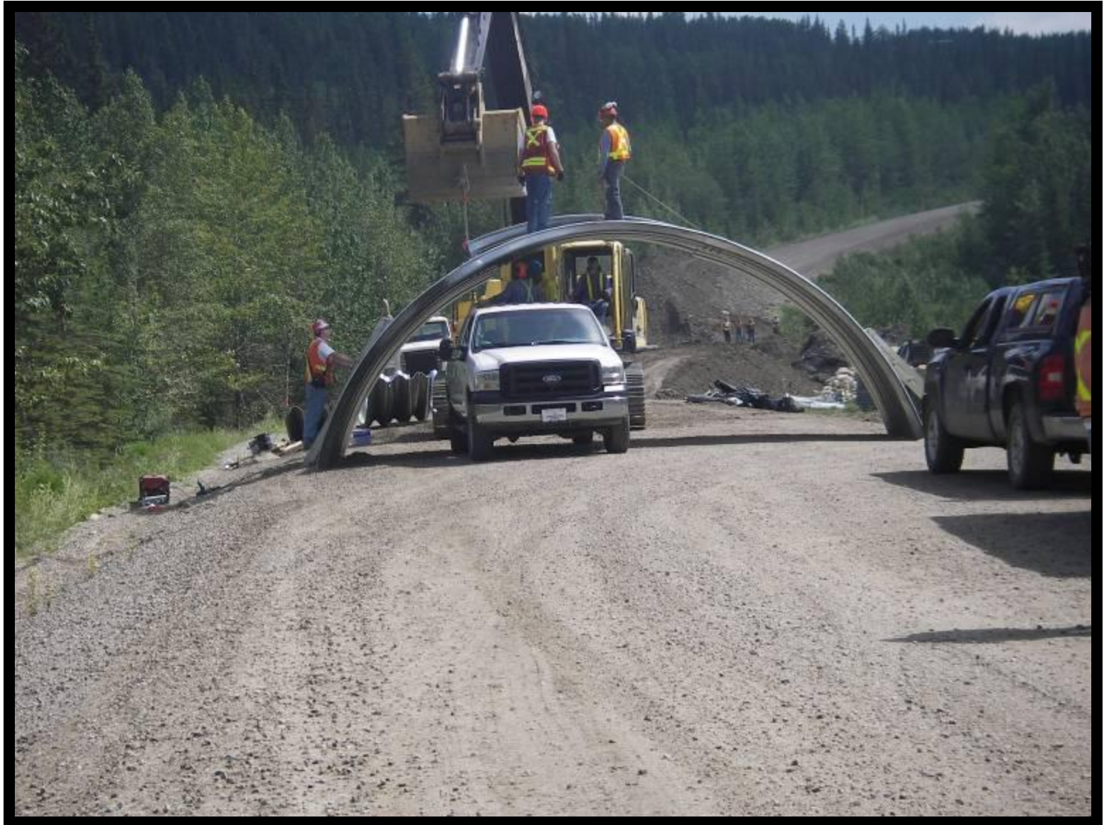
Construction of the metal arch before installation
