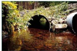
Properly installed culvert - photo courtesy of CulvertBC.com
