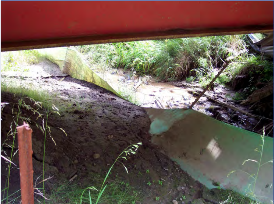
Road runoff-sourced sediment is spilling over silt fencing under bridge. Therefore, write “Yes” for evidence of sedimentation and “Road” or “External” for source of sediment.
