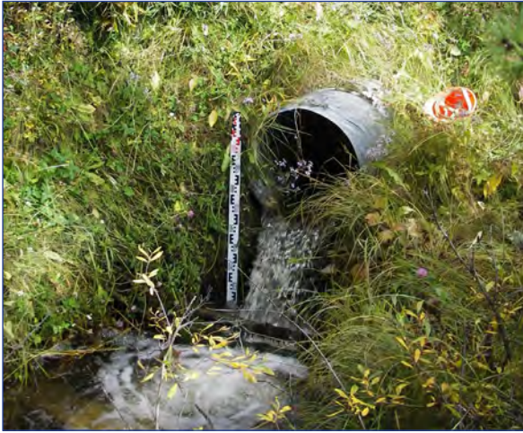
Hanging culverts present an obstacle to fish passage
