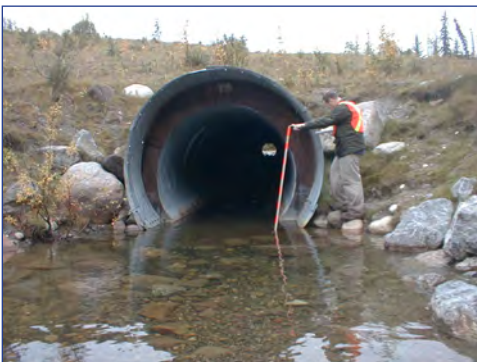
Backwater does not extend through entire culvert.
