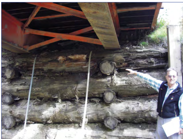
Structural problem (RA): Log abutment beginning to rot
