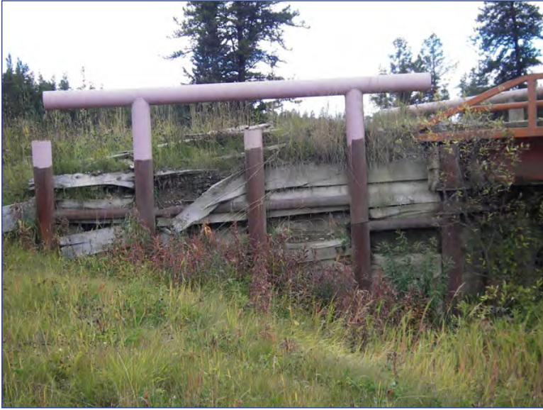
Structural problem (O): Pilings and rotted wingwall planks
