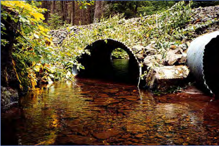
Properly installed culvert – photo courtesy of Culvert BC
