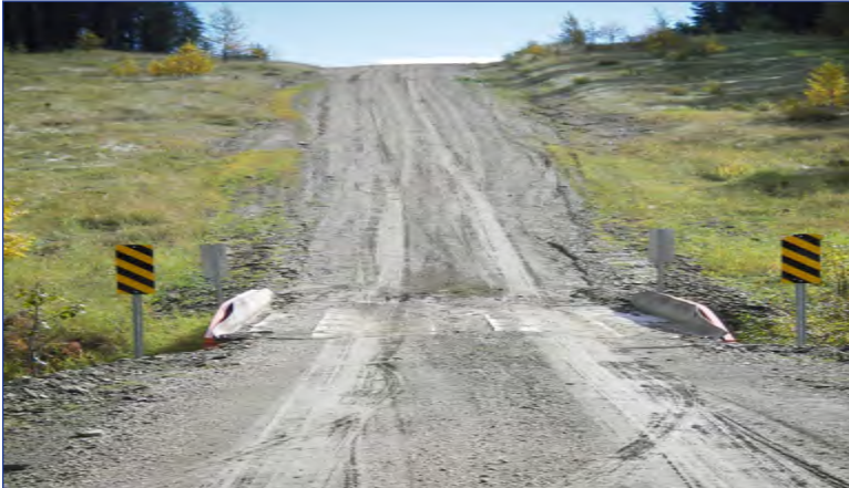
This bridge has geotextile curbs attached to the guardrail
