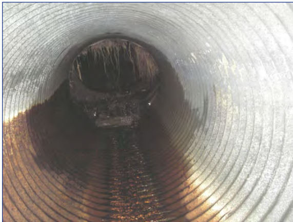
Structural problem (C): Culvert sections have separated, creating a sink hole above and dropping fill directly into the stream, and creating an additional barrier to fish passage
