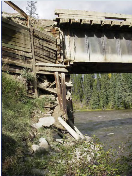
Treated wood wingwalls that are failing
