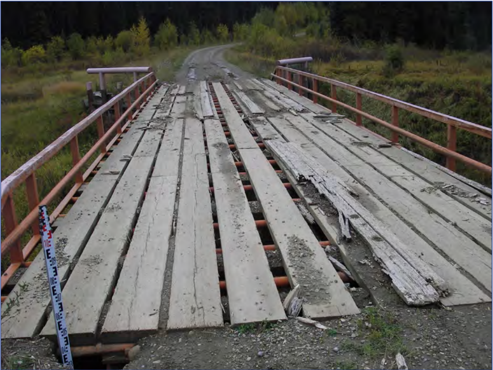
A large sinkhole near the bridge presents a high risk of an accident—emergency repair is warranted
