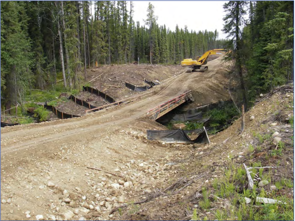
When used properly, silt fences are effective in controlling sedimentation during the revegetation period
