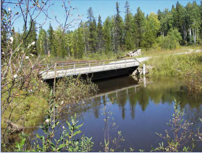
Upstream pond created by beaver dam blockage under bridge
