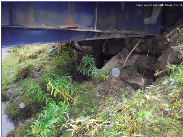
Structural problem (SL): Slumping caused by gully under bridge
