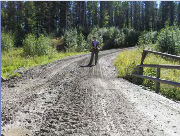
Structural problem (S): sunken deck
