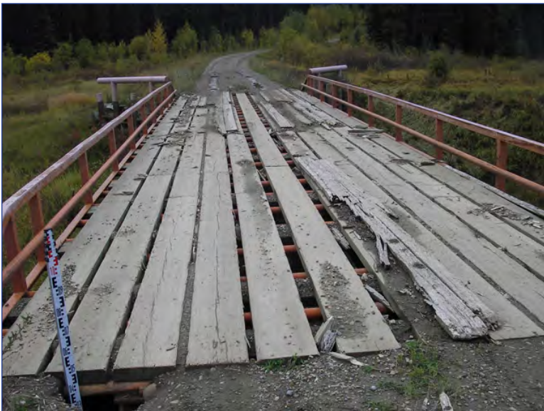
Structural problem (C): Collapsing causing sink hole
