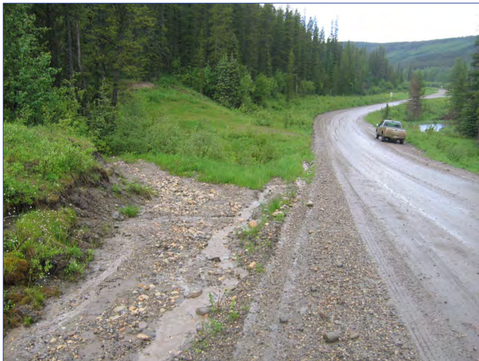
Blocked diversion ditch (requires Remedial Measures)
