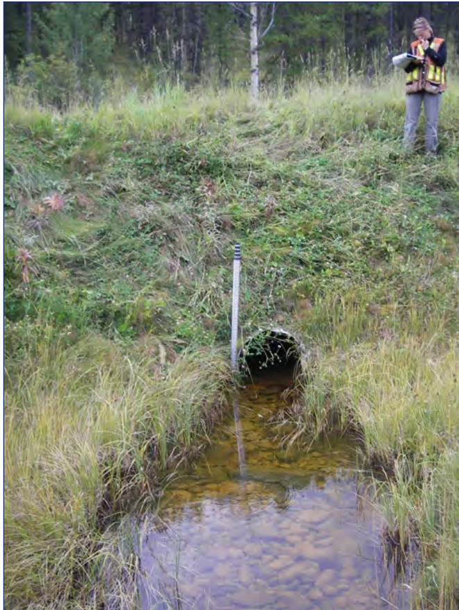
Vegetation is considered armour from an erosion perspective
