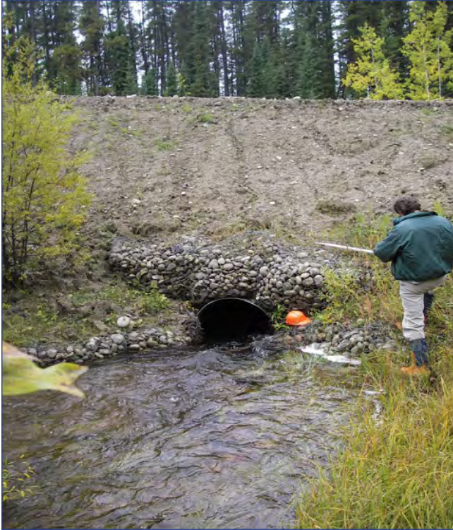
Gabion baskets used to armour the inflow. Note the rill erosion above the culvert
