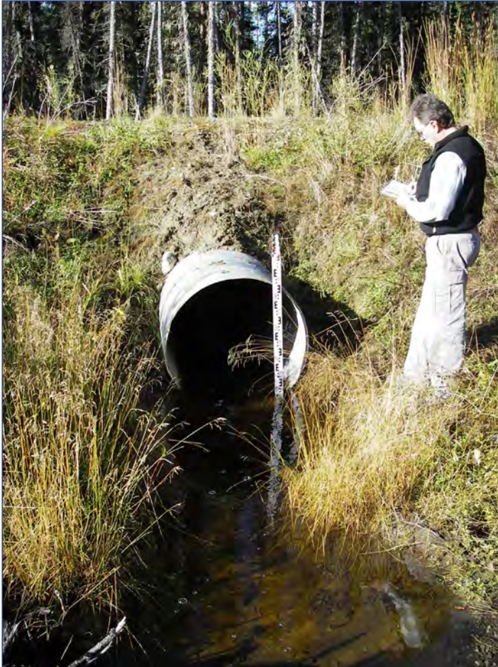
Round steel culvert
