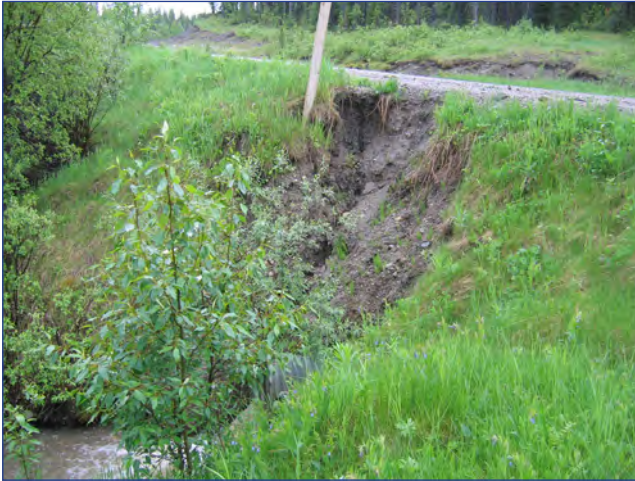
Fill slope erosion due to road surface runoff (requires Remedial Measures)
