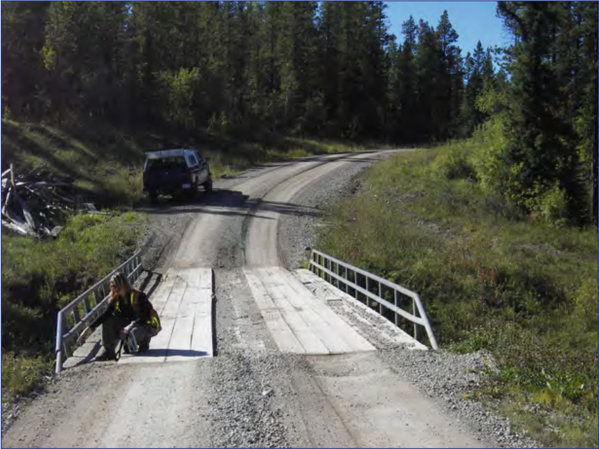
A closed decking pattern with no curb Note the broken guard rail.
