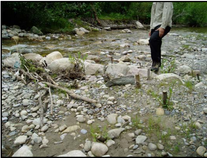
Photo: 25 Location: At Riffle 4 View: Downstream from RDB Description: Live staking at root of Riffle 4
