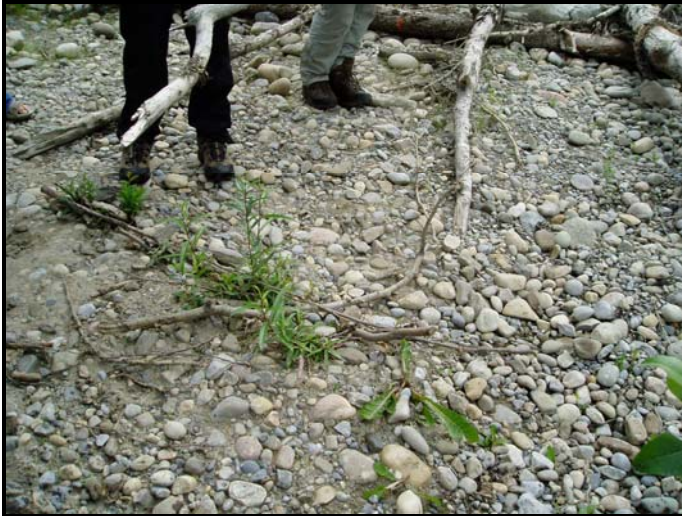
Photo: 1 Location: Below Riffle 9 on RDB View: Upstream Description: Successful live stakings
