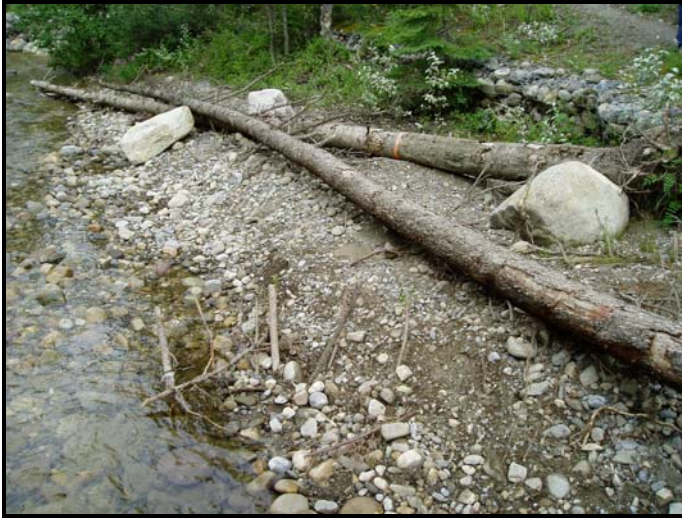
Photo: 13 Location: Above Riffle 7 View: Downstream from RDB Description: LWD anchored to bed on RDB
