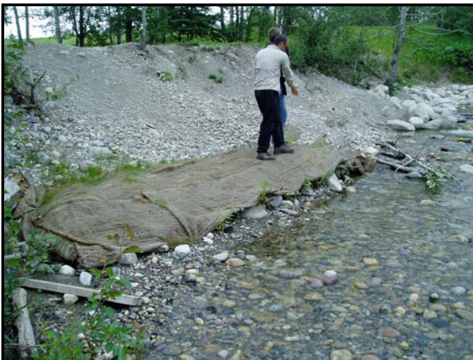
Photo: 36 Location: Below Riffle 1 View: Upstream Description: RDB bank treatment below Riffle 1
