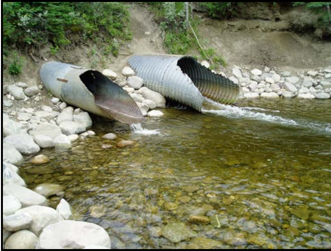
Photo: 40 Location: At Hardisty Avenue View: From RDB Description: Hardisty Avenue culvert outlets
