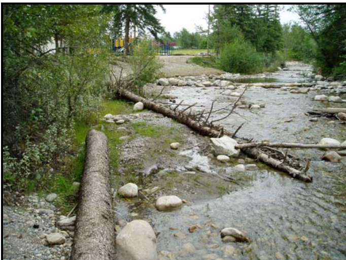
Photo: 27 Location: Above Riffle 4 View: Upstream Description: LWD anchored to bed on RDB above Riffle 4
