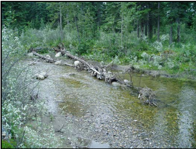
Photo: 14 Location: Above Riffle 7 View: Upstream from RDB Description: LWD anchored to bed on LDB
