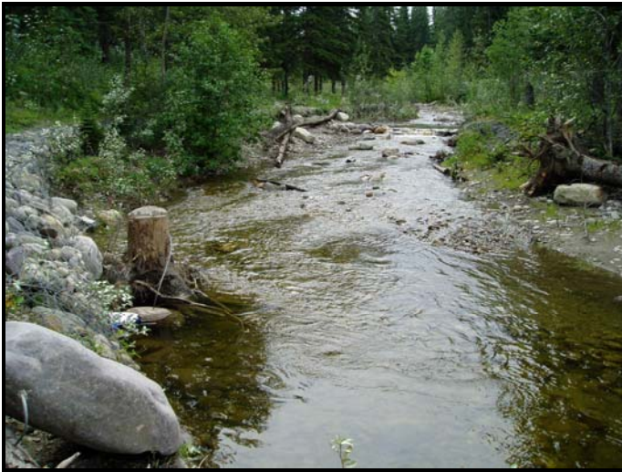
Photo: 10 Location: Above Riffle 8 View: Upstream Description: LWD (root wad) anchored to RDB above Riffle 8
