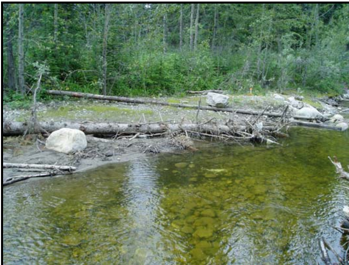
Photo: 9 Location: Above Riffle 8 View: From LDB Description: LWD anchored to bed on RDB, note sediment deposition at upstream end
