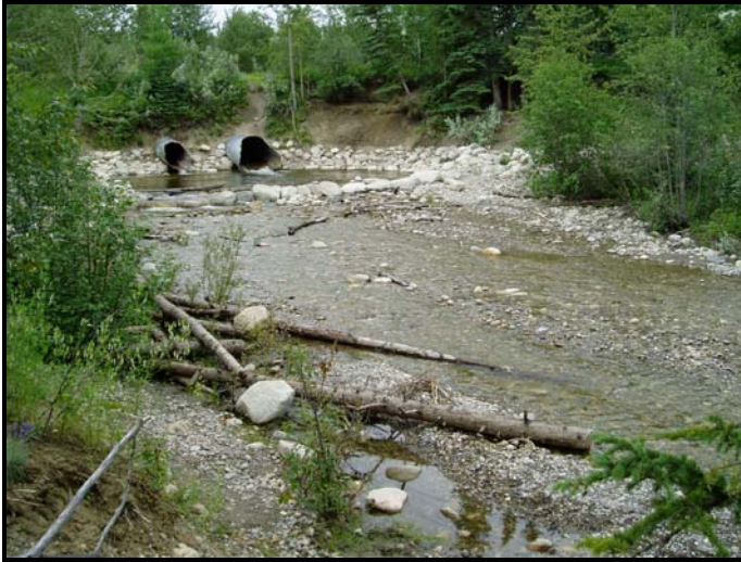
Photo: 34 Location: Below Riffle 1 View: Upstream Description: LWD anchored to RDB below Riffle 1
