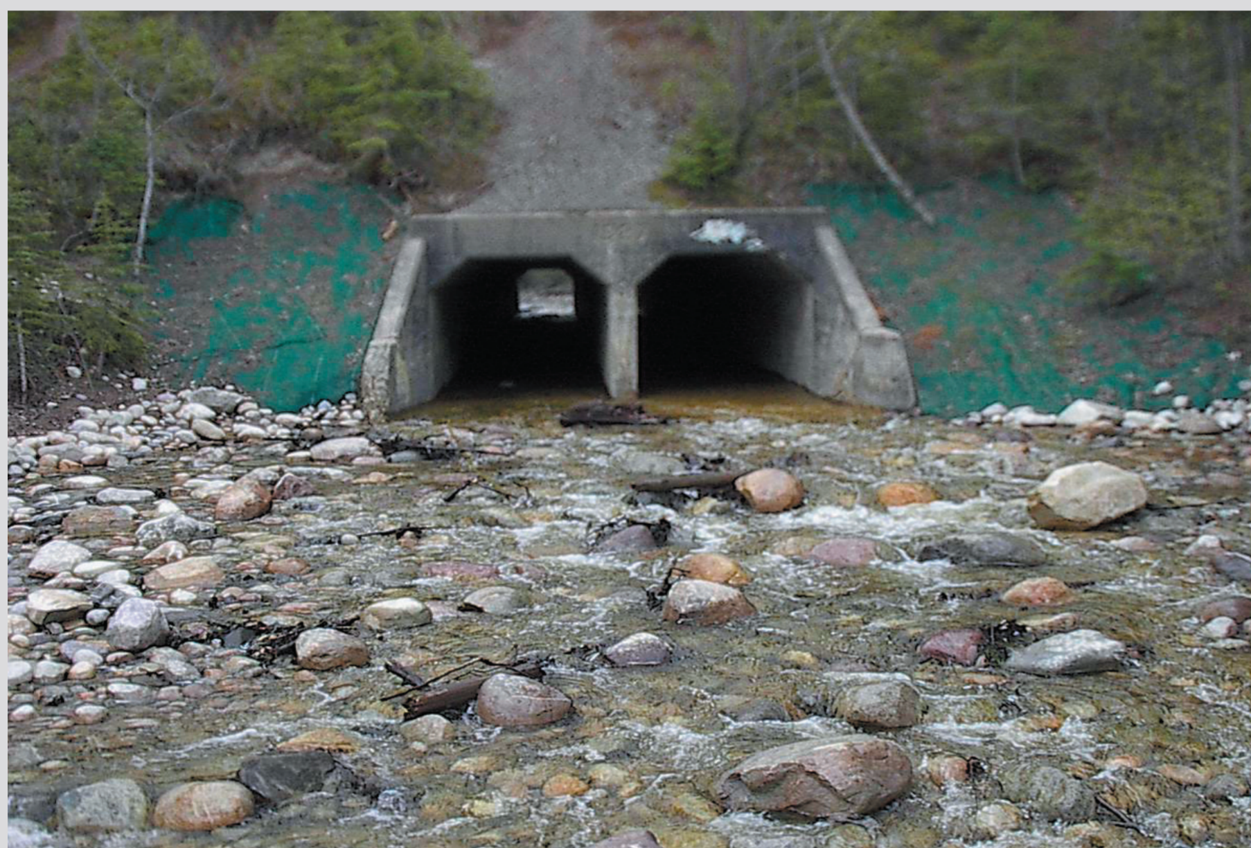
Canadian National Railways stream crossing after restoration work was completed in 2003.
