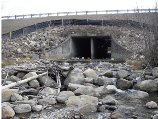
Hanging culverts at reach end.
