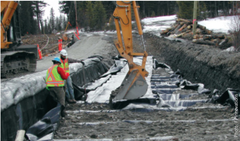
Fig. 2: Geotextile laid across pile caps is backfilled to form the GRS base.
