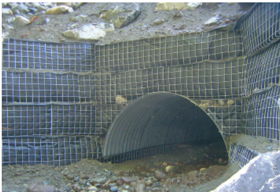
Fig. 1: Outlet of GRS open-bottomed arch founded on in-situ soils.
