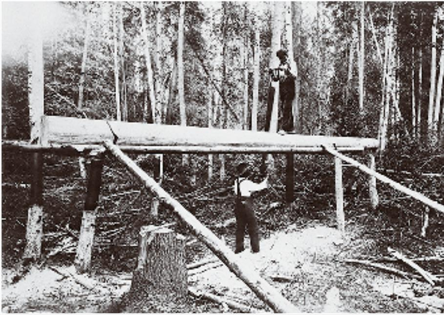
*Whip Sawing Lumber on Lake Linderman, 1898. This system was widely used where a lumber supply was needed and no sawmills or transportation was available. While the man on top worked harder, the man below was considered to have the worst job, “eating” sawdust with every saw pull. Jack Glen made lumber for the Mile 58 cabin this way.*
