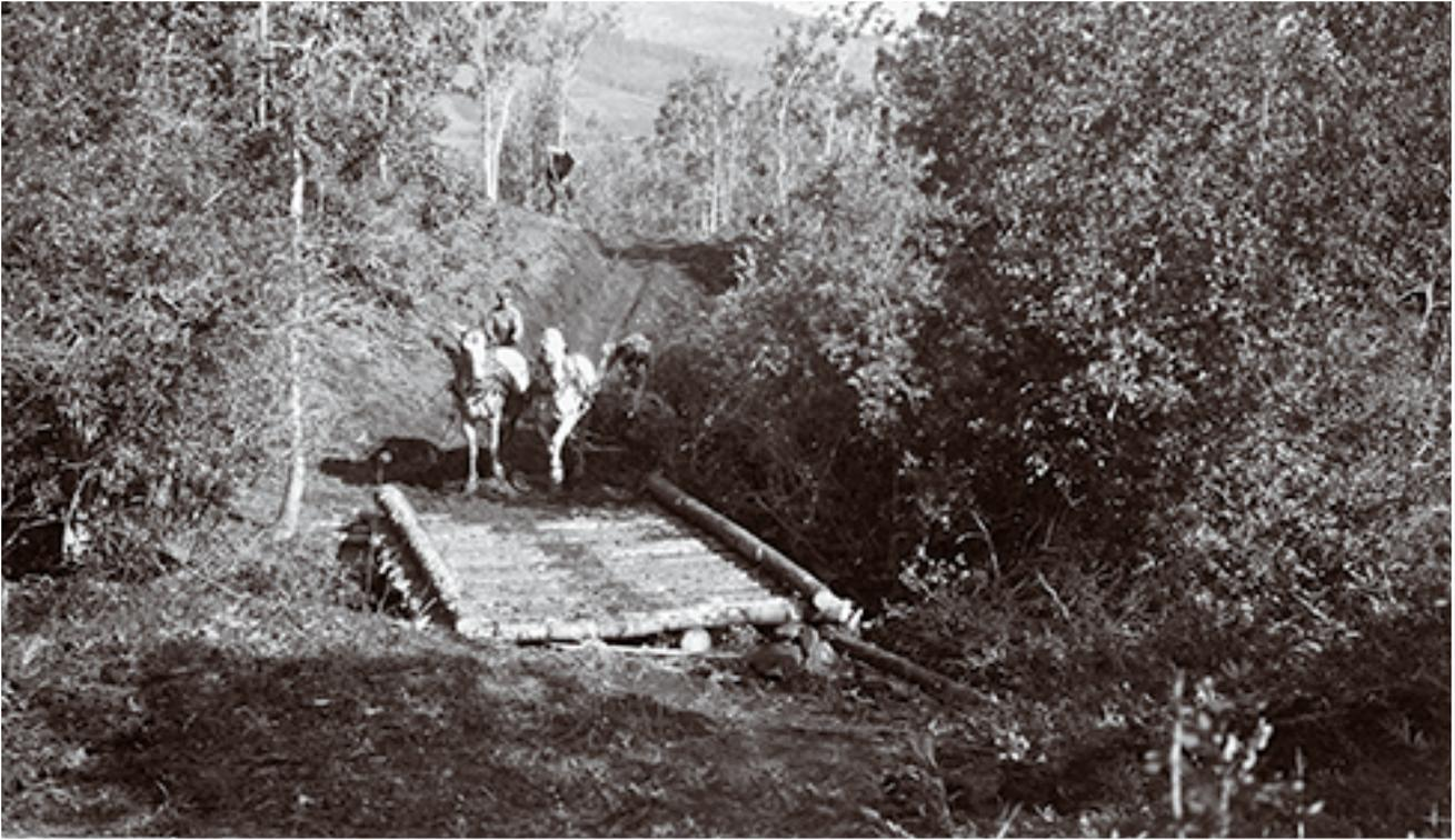
*The early Forestry bridges, such as the ones across the Wildhay and Berland Rivers, were typically built of local timber with log abutments and rock-filled cribs to support longer spans. The bridge in this photo is on the Highwood-Pekisko Creek road in the Bow River Forest, 1923.*
