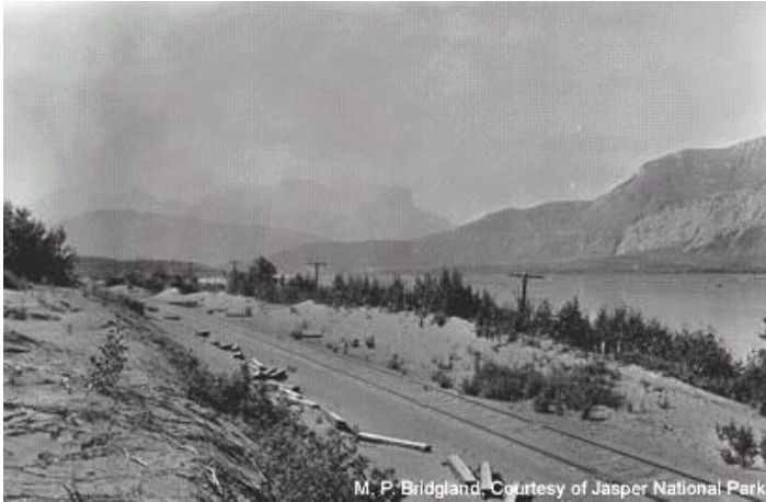
Newly-Constructed GTP RR Line Already being Buried by sand. Brule Lake, 1915. Photo credit: M.P. Bridgland DLS
