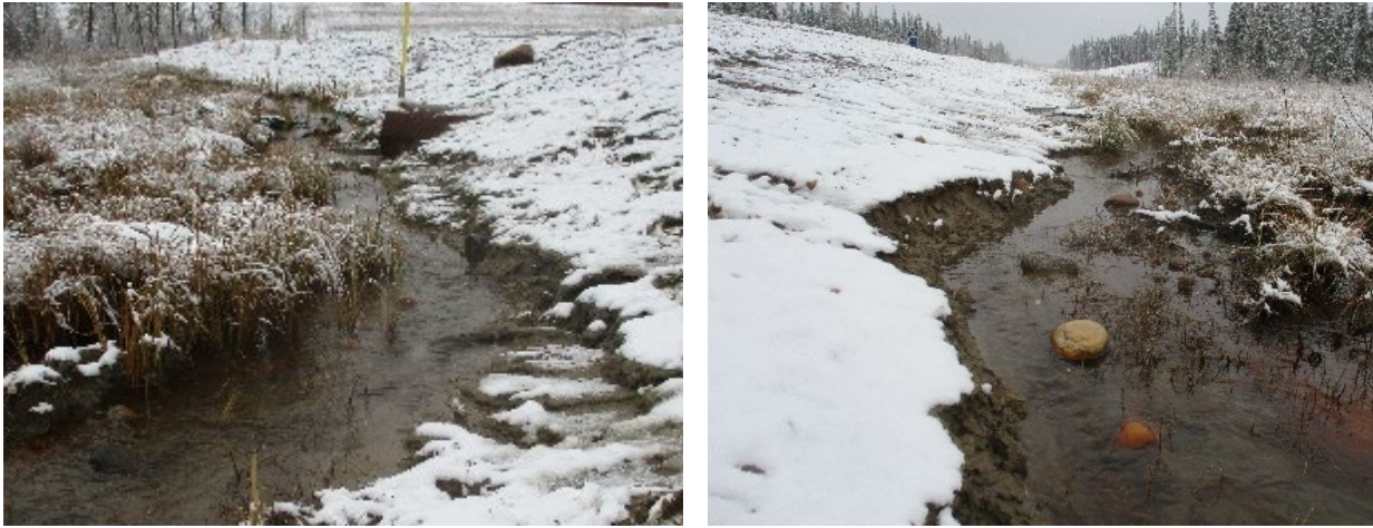
Figure A6. Wetland flow along the road embankment moving towards the nearest downslope conduit can flow with enough energy to erode both deposited sediment and the lower road embankment. In this case the sediment produced from the road embankment was re-suspended from its initial deposition location (right and left photo are the same site in opposite directions), meaning that the initial deposition area may therefore not be the only or final receiving environment.
