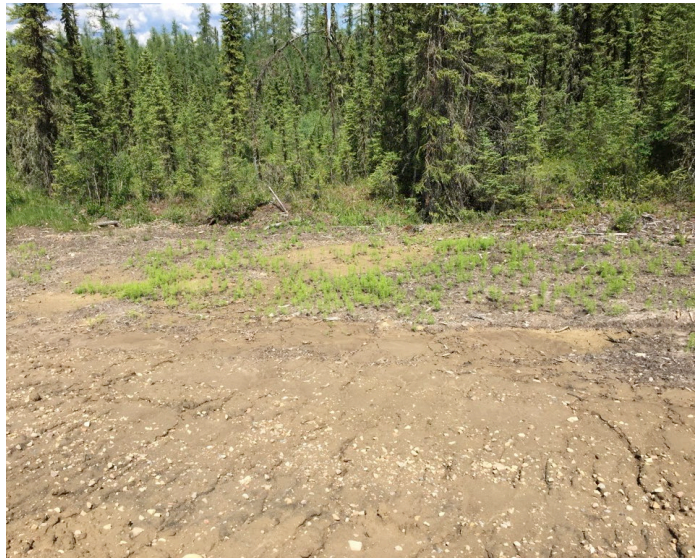
Figure 15. Road erosion delivering sediment into peatland. Road fill may cause nutrient loading and alter peatland chemistry, thereby changing the environment and affecting the habitat of peatland plants and animals (e.g., amphibians).
