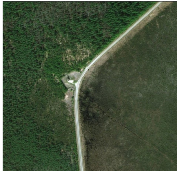
Figure 12. Marked differences in vegetation height and colour and pooling of water on one side of the road are indicators of flow impediments at this crossing. Image courtesy of DUC.
