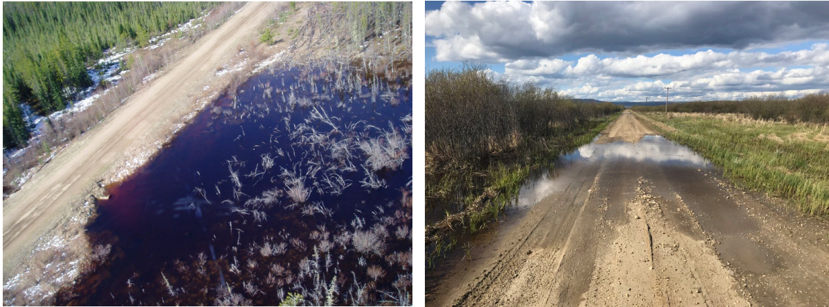
Figure 7. Examples of problems at wetland crossings likely related to hydrologic disruption. Left: flooding on one side of road, causing die-off of vegetation and potential development of an open water wetland. Right: flooding over top of road, likely leading to saturation of the road base and increasing proneness to rutting; differences in vegetation on either side of road also suggest that wetland flow may be impeded.
