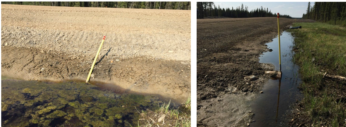
Figure A7. Sunken culvert (left) is not problematic if it is not plugged, as it will drain subsurface flow. Righthand photo is outlet of the same culvert. It may actually be desirable to install culverts in pairs separated by a distance of 10 m or so, with one culvert below the surface and one embedded 20-30%.
