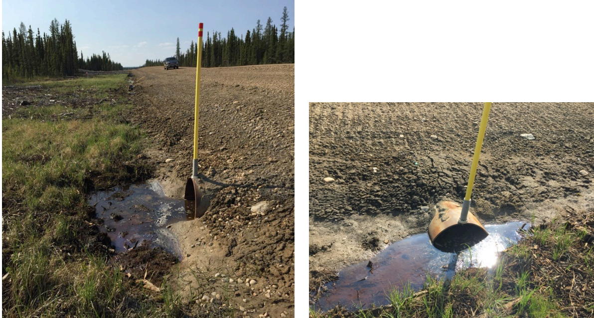
Figure A1. Well-functioning culvert crossing a peatland. Left: culvert inlet is embedded about 50% compared to the original peatland grade. A trench was dug into the peat and the culvert installed on piles within it. The open water area in front of the culvert is the end of the trench. Notice that the water level is below the peat surface. This culvert is functioning well by draining both surface and subsurface flow and delivering it to the other side of the road, preventing upwelling of the subsurface flow. Right: culvert outlet.
