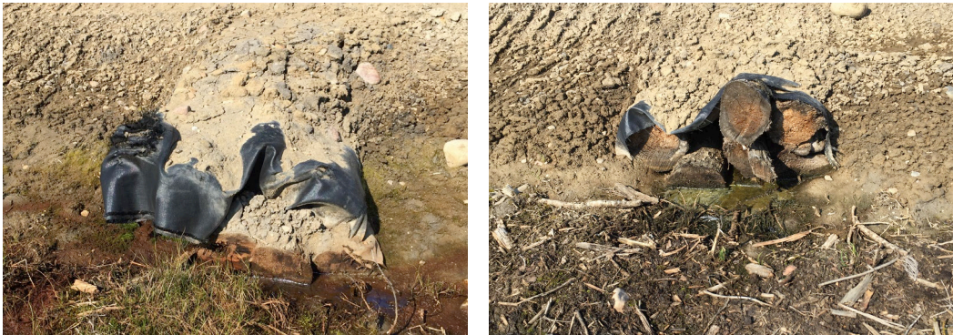
Figure A4. Erosion/sedimentation around log bundles may negatively impact water quality of the surrounding wetland. Left: erosion and sediment possibly impeding water flow through a log bundle. Geo-fabric also potentially impeding flow. However, the fabric on top of the logs is also preventing the voids between logs from becoming clogged by sediment. Right: logs should be embedded into the peat as shown to allow for continuous subsurface flow, but sedimentation should be controlled.
