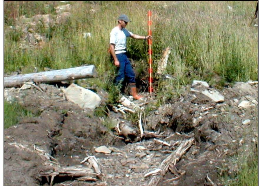
Figure 4. A reclaimed road crossing at an intermittent stream with a gully terminating in an 80cm headcut. Although intermittent streams may be so small they are unmapped, post-fire runoff can be sufficient to scour the un-vegetated portion of reclaimed road crossings.
