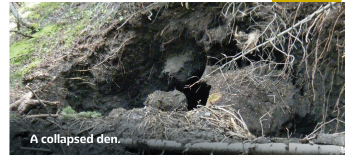
Dens can look like erosion and can be found along riparian slopes.
