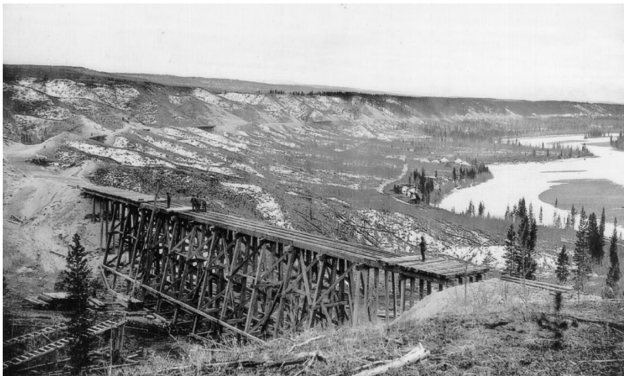
Canadian Northern Railway construction east of Hinton ca. 1912-13, below the Obed Hills looking westerly. The railway construction tent camp is along the river.
