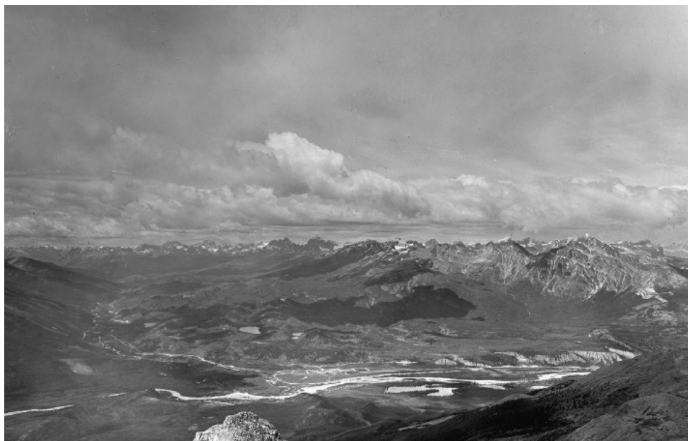
View westerly up the Miette River across its junction with the Athabasca River above Jasper, the route to the Yellowhead Pass. Photo by M.P. Bridgland from Mount Tekarra in 1915. Clearings show the location of the recently completed Grand Trunk Pacific Railway and site for the future town of Jasper.
