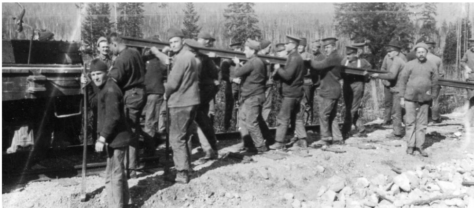
Lifting steel from the abandoned railway line near Red Pass intended for the First World War effort, ca. 1917.
